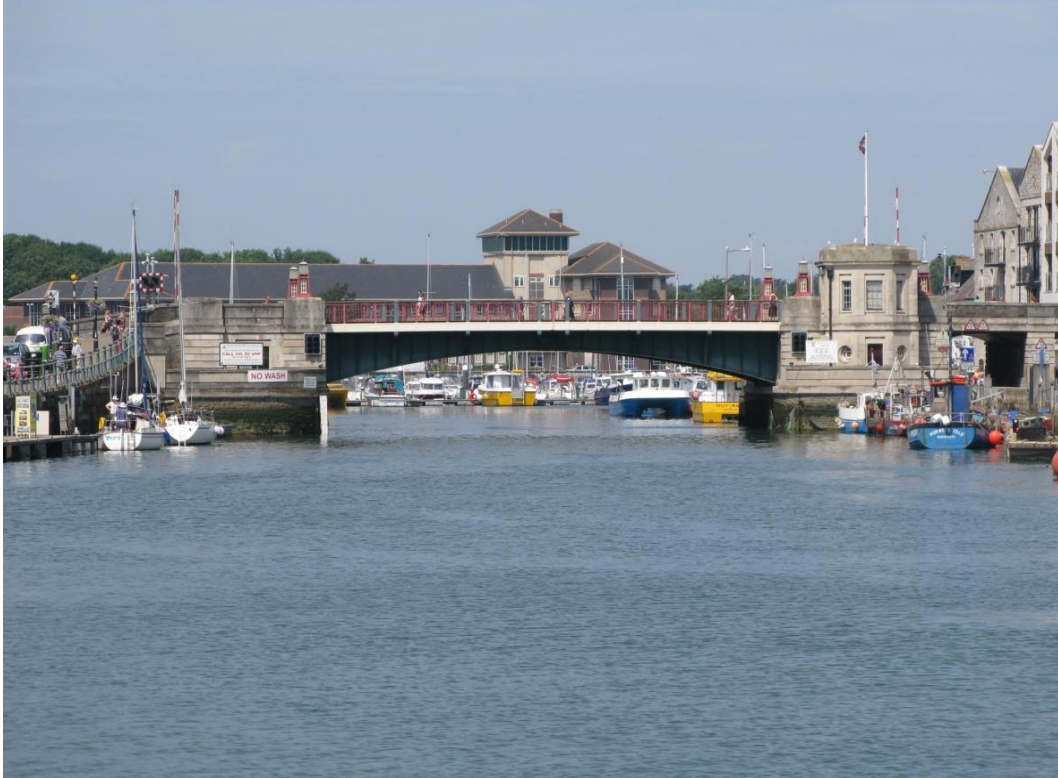
Figure 3. Town Bridge closed
